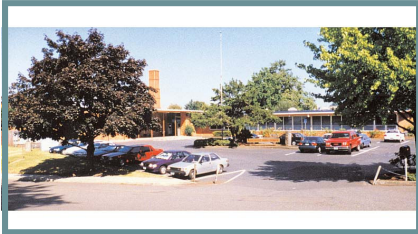
West Sylvan Middle School 8111 SW West Slope Drive Portland, OR 97225
